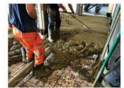
installation time, which means that one person can lay Orlitech mesh some three times faster than traditional steel mesh. Health and safety risks are reduced due to the lightweight 0.35kg/m² and ease of cutting. All these characteristics contribute to great financial savings."
